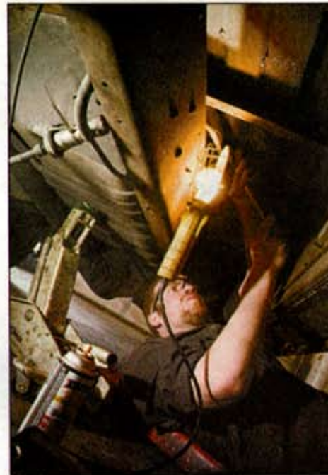
Golden Fuel Systems' John Grant unbolts a fuel tank on a conversion van to install a custom-made unit necessary for the diesel engine to run on vegetable oil.
